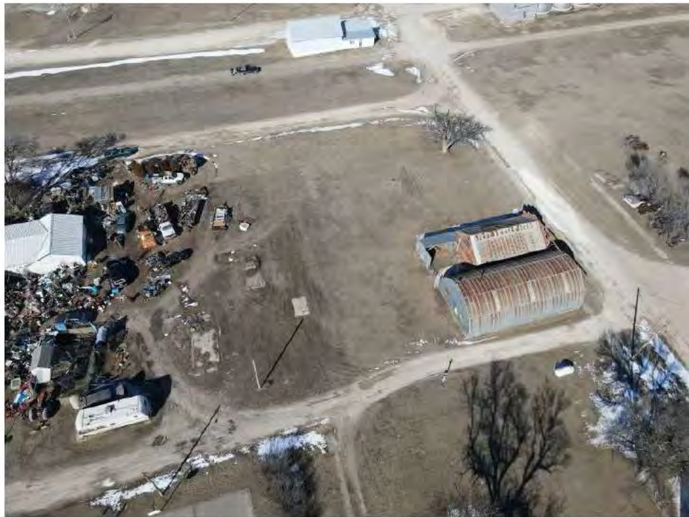
BELOW: Aerial Photo facing North
